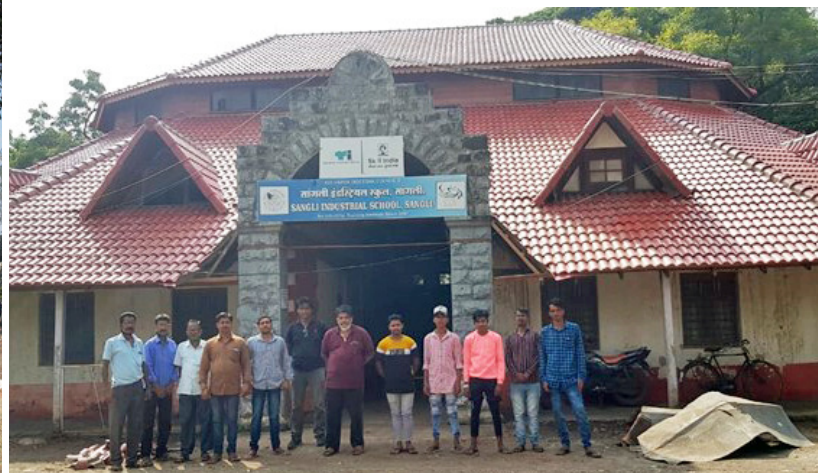
Sangli Industrial School after renovation
